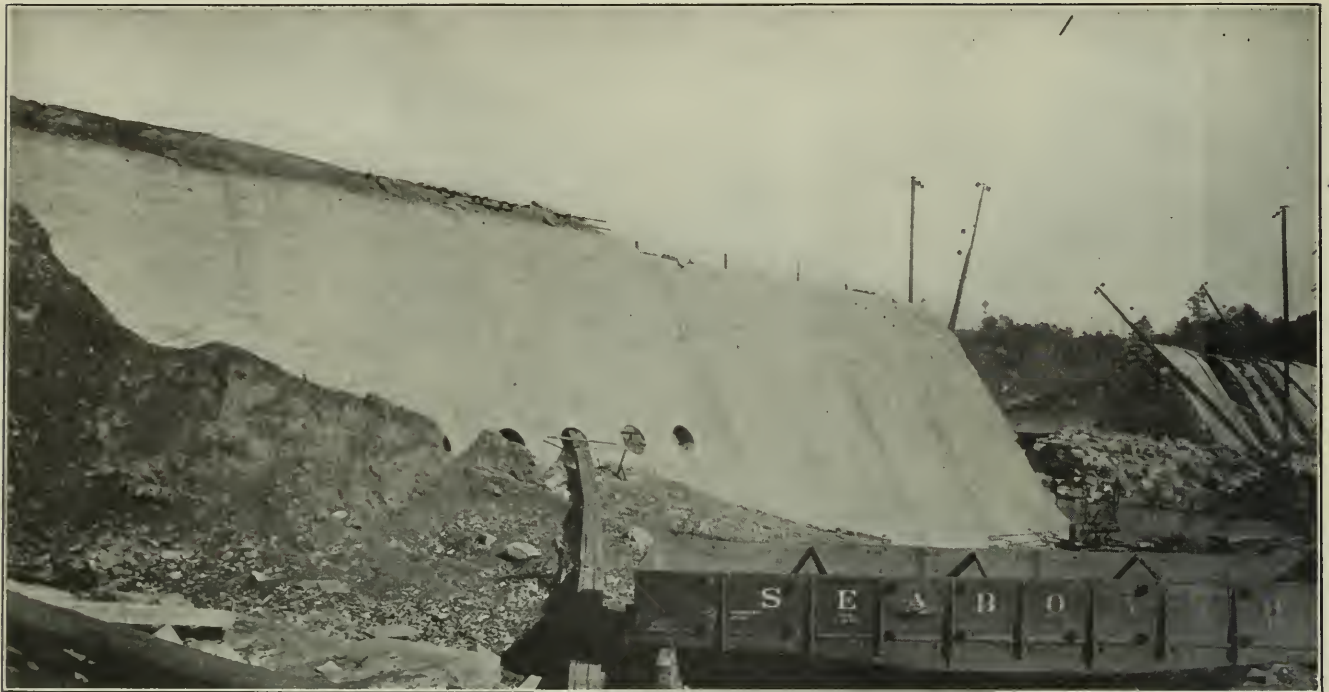
FIG. 5. THE ROCKY CREEK DAM DURING CONSTRUCTION
